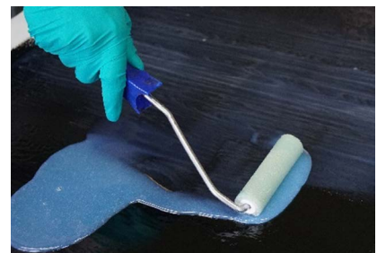
Roller application of SikaBiresin CR169 thix
