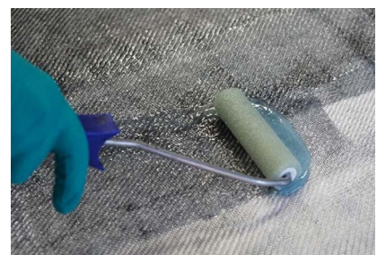
Wet lay-up with SikaBiresin CR168
